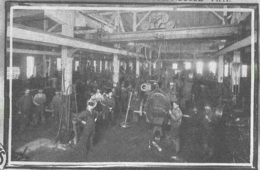
ENGINE ERECTION SHOP.
