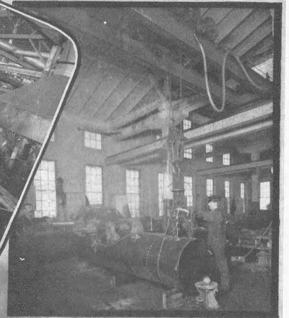
DRILLING BOILER WITH COMPRESSED AIR.
