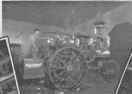
16-HORSE ENGINE DOING 39-HORSE POWER WORK UNDER FRICTION BRAKE
